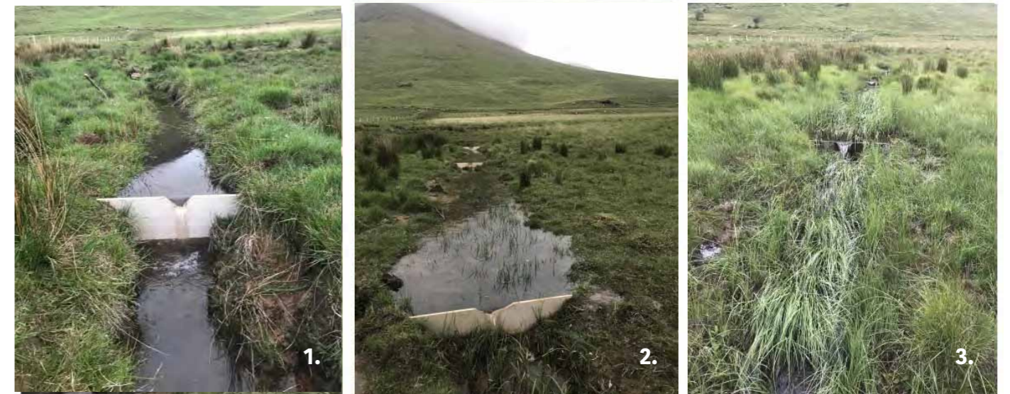
Figure 9. Drain-blocking measures completed in spring 2020 with rapid recovery of vegetation that reactivates important wet flush areas that reduces silt loads to the river.
